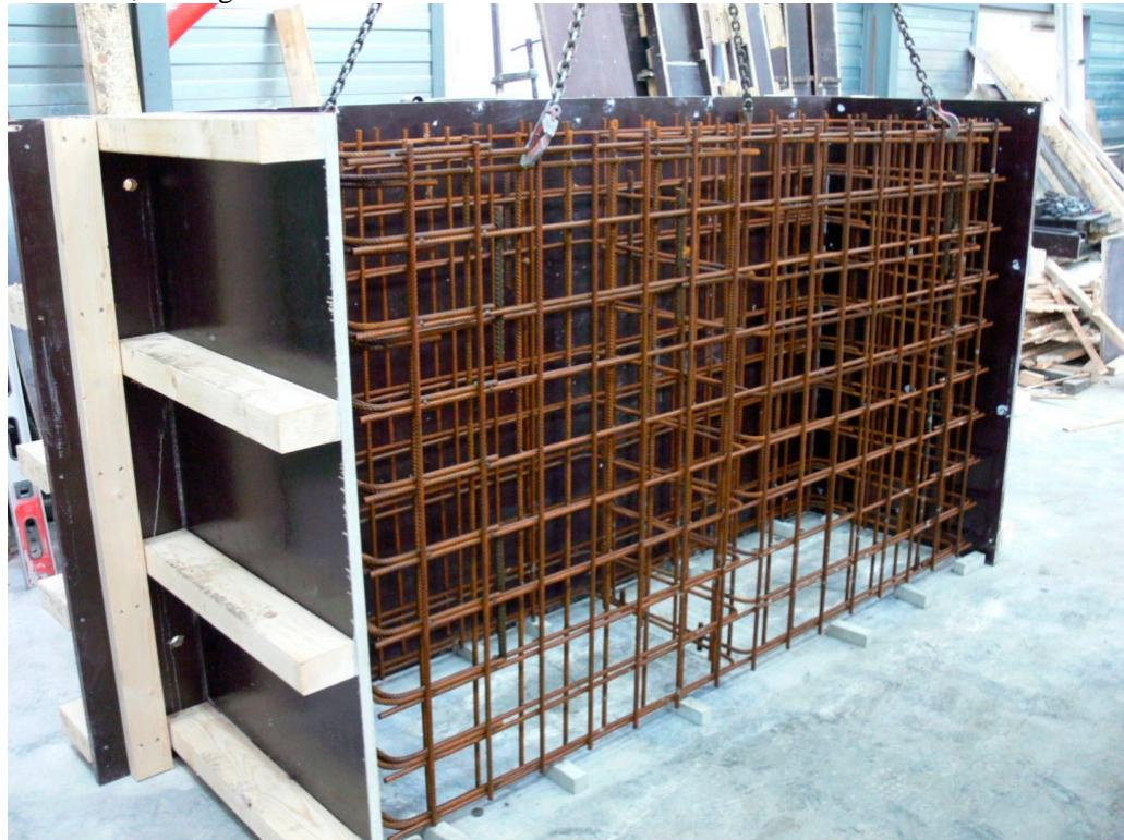
Figure 3.2 Mould for the casting the elements with the reinforcement in place
